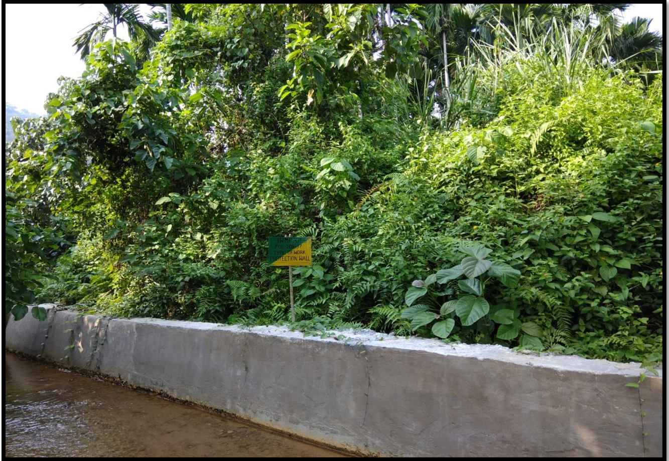
Protection Wall of Shri. Arbis Tangdhara at Tharia, Wah Mawblei Watershed.
